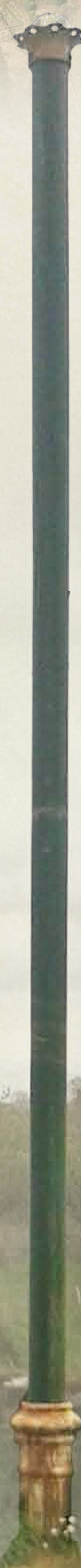
Sewer ventilation pipe, Maugheraboy
